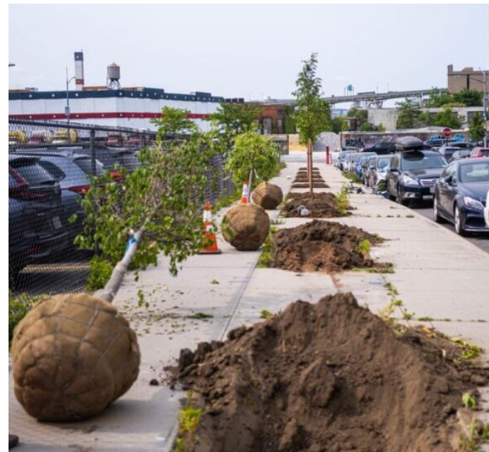
Balled and burlapped trees being planted in Long Island City, 2023. Photo credit: Haley Hix, NYC Parks
